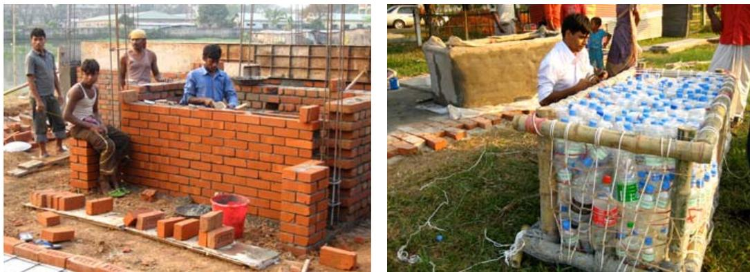
Figure 7: The LIFT House in Dhaka, Bangladesh. Concrete and brick base structure under construction; buoyancy block made of recapped, recycled plastic bottles.
