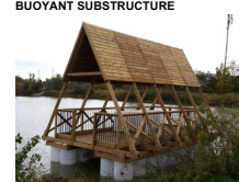
PAVILION AS INSTALLED ON THE UWATERLOO CAMPUS IN 2018
