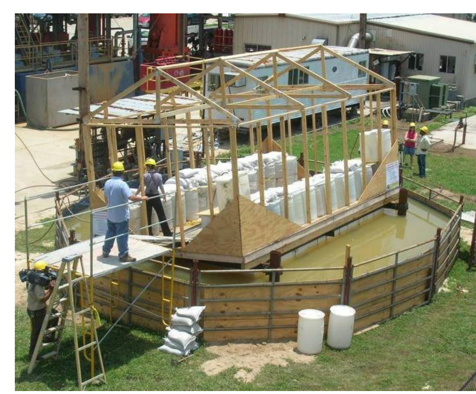
MOVING SANDBAGS TO TILT THE HOUSE
