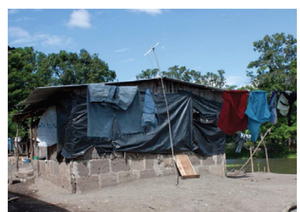
EXISTING HOME IN MALACATOYA
