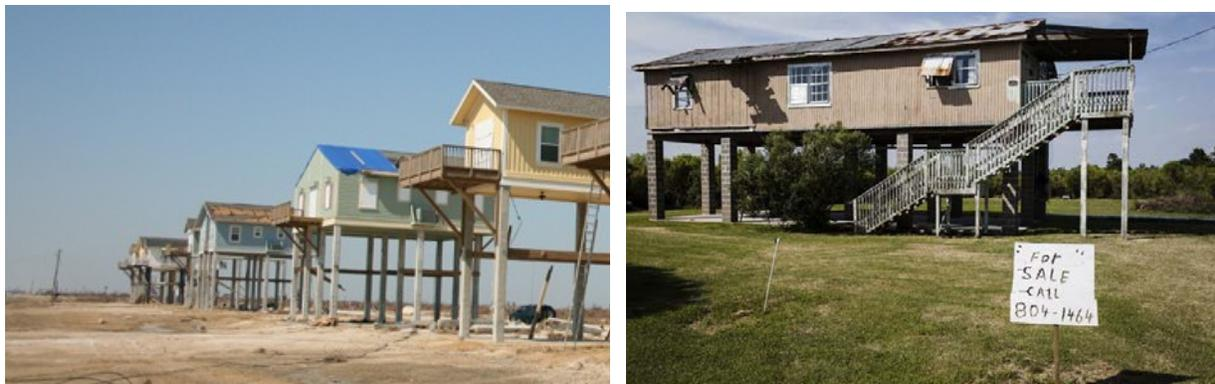
**Figure 1.** Increased exposure to wind with permanent static elevation
