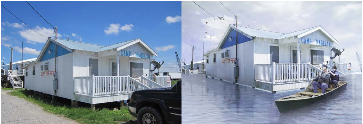
Fig. 5. (a) Current house conditions; (b) Render of elevated house during flood after installation of a Buoyant Foundation (Author: Ivey Wang, University of Waterloo)
