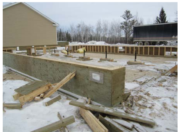
Figure 6. (a) existing manufactured homes on military base; (b) pony-wall foundation system for existing manufactured homes
