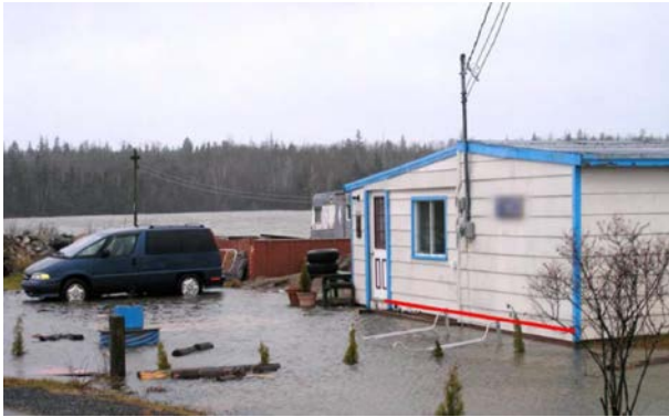
Figure 4. Original Cow Bay Cottage (static structure) in mild flood condition.
