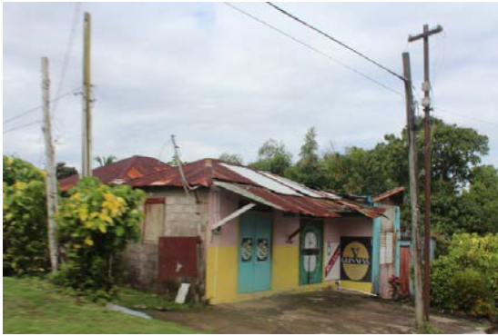
Fig. 3. concrete masonry unit structure on concrete slab (photo credit: Scott Turner)
