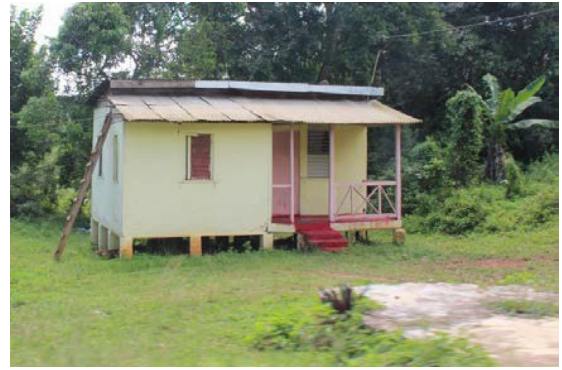
Fig. 4. wood frame structure on pier-and-beam platform (photo credit: Scott Turner)
