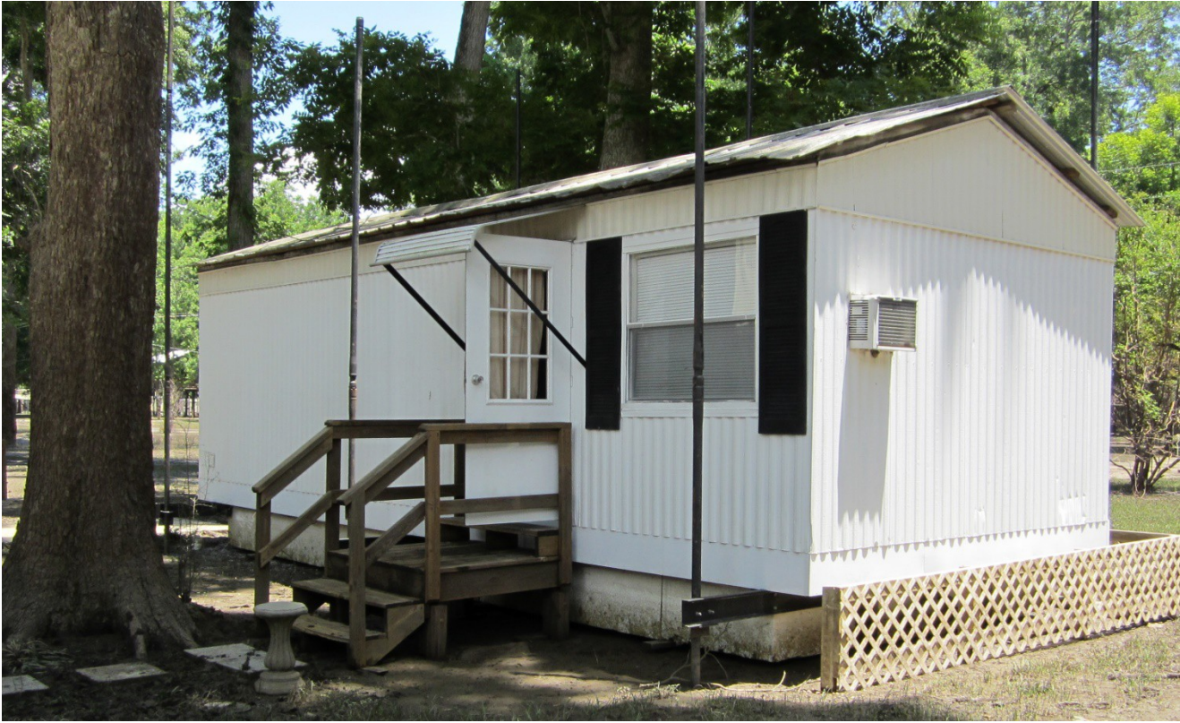
Fig. 2-House in Old River Landing, Pointe Coupee, Louisiana, USA with amphibious foundation (photo credit: Elizabeth English)
