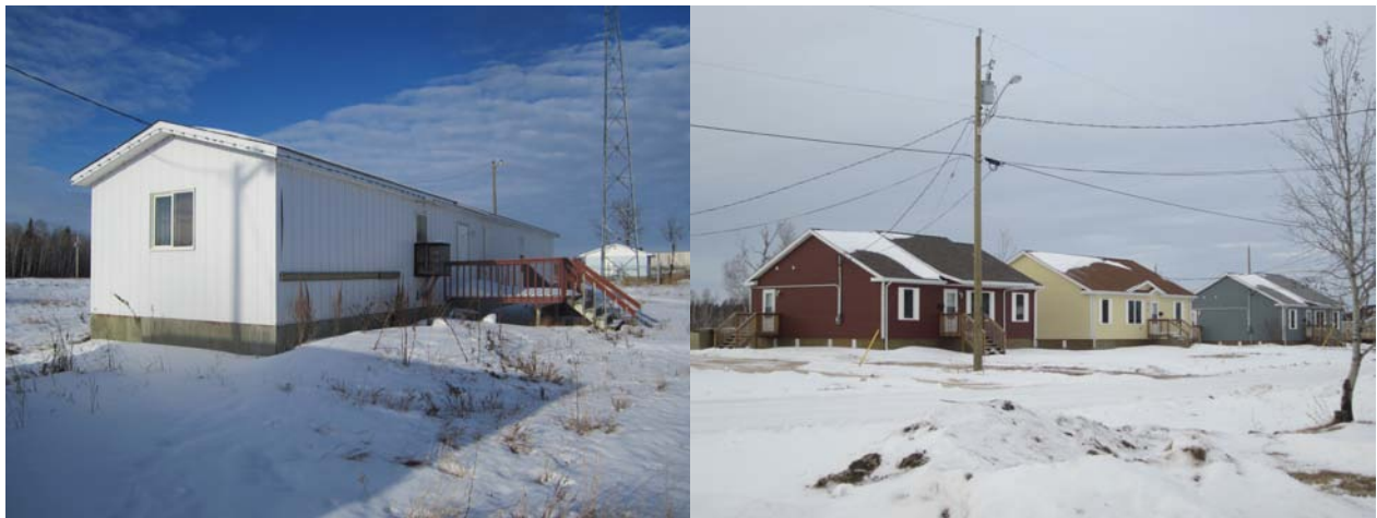
Fig 5. (a & b) Prefabricated homes on the Pinaymootang reserve, representative of housing types common to the area that could be retrofitted with buoyant foundations.
