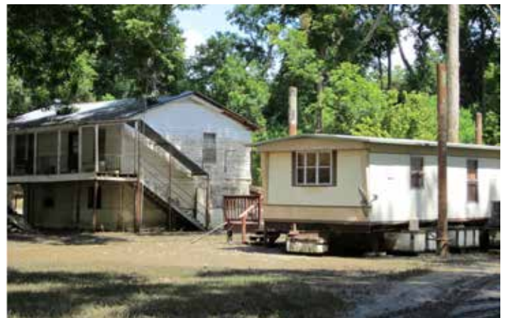
FLOOD DAMAGE WITH STATIC ELEVATION VS. AMPHIBIOUS
