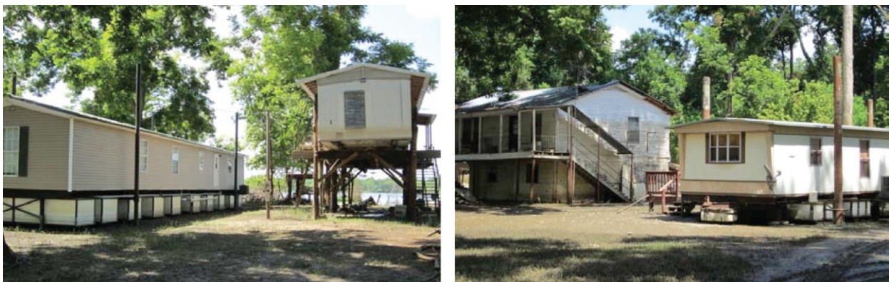
Fig. 4 Comparison of flood performance of amphibious houses (undamaged) vs. PSE structures (damaged), Old River Landing, Louisiana (photos permission of Buoyant Foundation Project)
