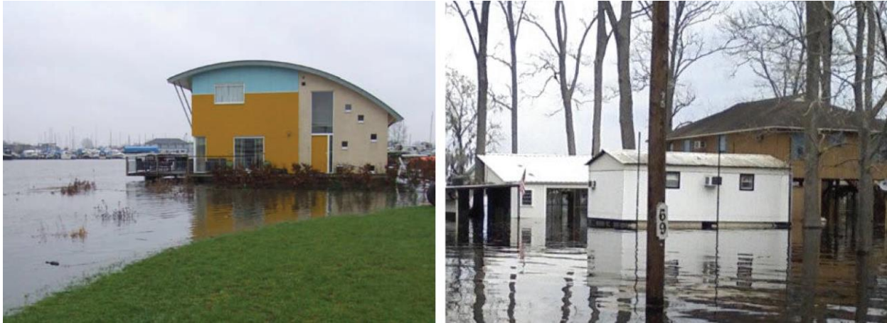
Fig. 3 Flood performance of amphibious houses in Maasbommel, The Netherlands, and Old River Landing, Louisiana (photos permission of Buoyant Foundation Project)
