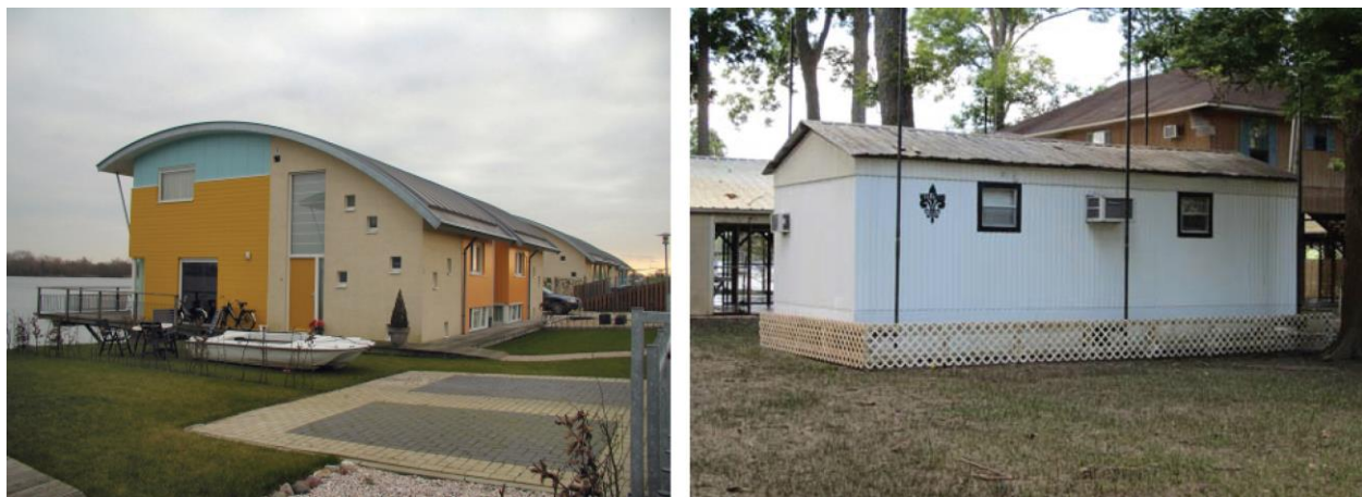
Fig. 2 Amphibious houses in Maasbommel, The Netherlands, and Old River Landing, Louisiana (photos permission of Buoyant Foundation Project)
